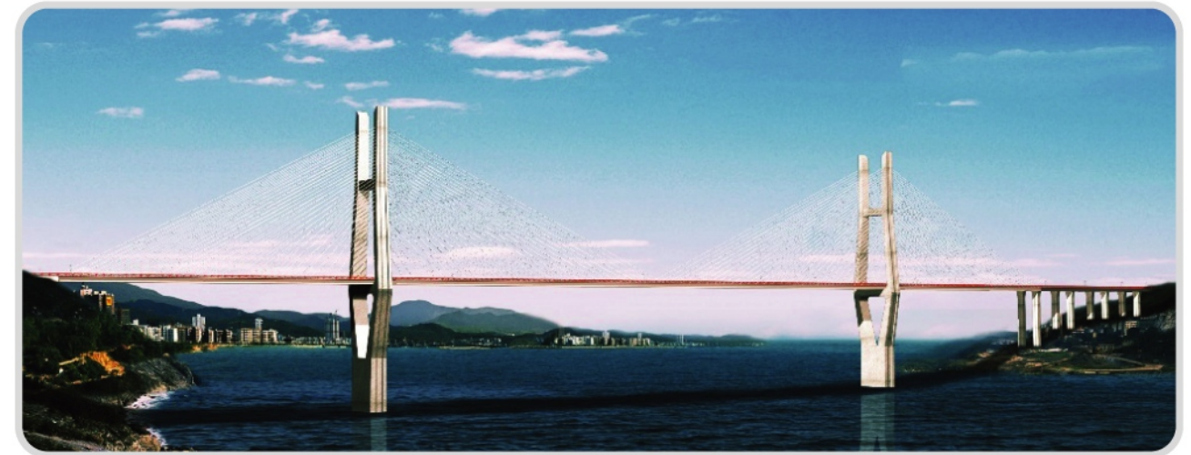
④ Lidu Yangtze River Bridge in Poling Chongqing ● Size and Quantity: 7x109 ~ 265, totally 10 sizes
