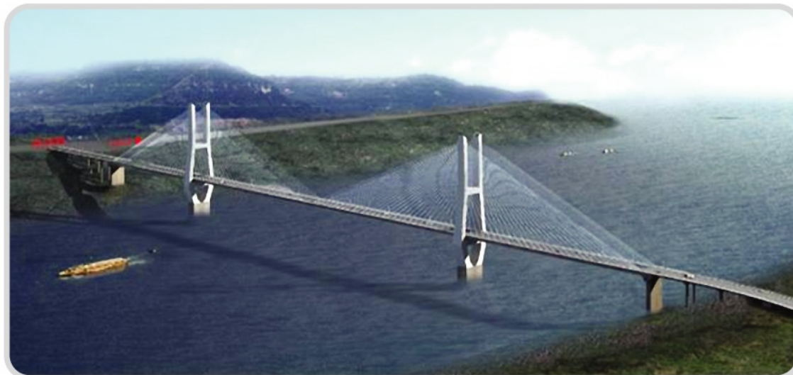
④ The Yangtze River Highway Bridge in Changshou Chongqing ● Size and Quantity: 7x127 ~ 283, totally 7 sizes
