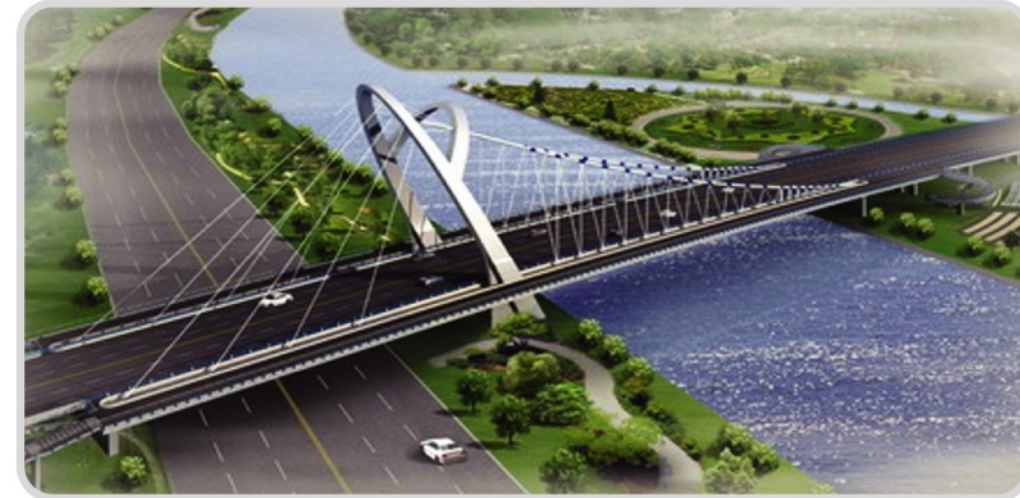
📍 Changzhou Longcheng Bridge ● Size and Quantity: Main Cable Strand 7x397, span 110m, Back-Stayed Cable 7x253, Lifting Rod 7x73
