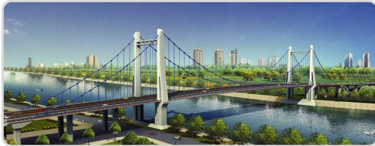
📍 Ningbo Qingfeng Bridge ● Size and Quantity: Main Cable Strand 37 - 5.1x91, span 280m, Lifting Rod 5x91, 5x121
