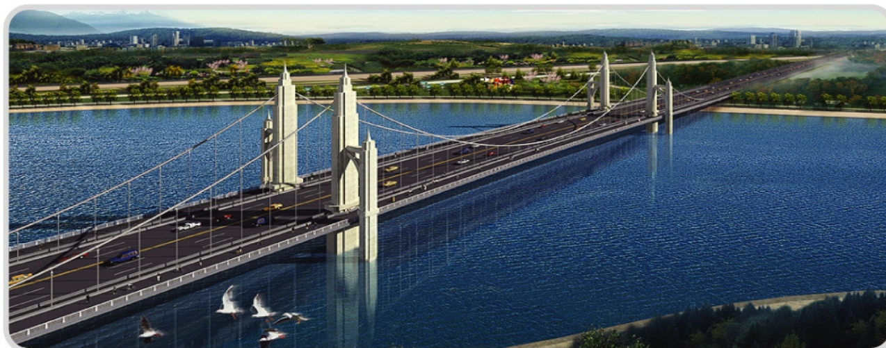
📍 Beijing Changping South Circle Road Bridge ● Size and Quantity: Main Cable Strand 19 - 5.4x127, span 177m, Lifting Rod 7x73
