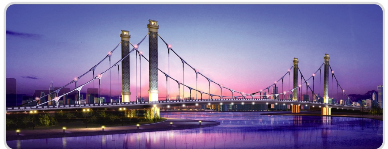
📍 Qin Zhou Zicai Bridge ● Size and Quantity: Main Cable Strand 37 - \phi 5.3x127, span 158m, Lifting Cable \phi 7x121, \phi 250 rigid lifting rod
